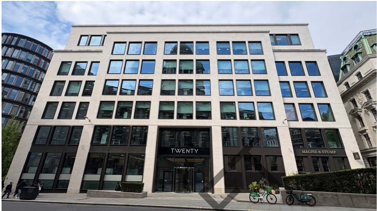
Photograph 1 – General view of the front east elevation constructed in 2017.
