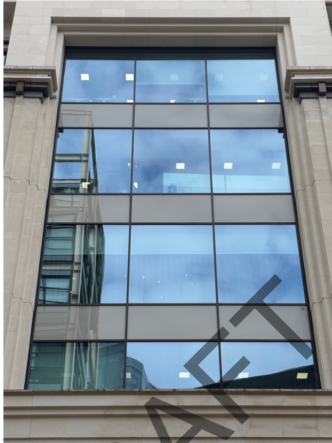
Photograph 11 – West elevation 2017 curtain wall over entrance.
