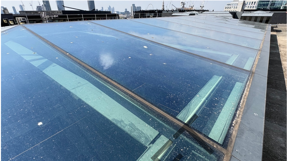
Photograph 17 – General view of the glazed atrium roof.
