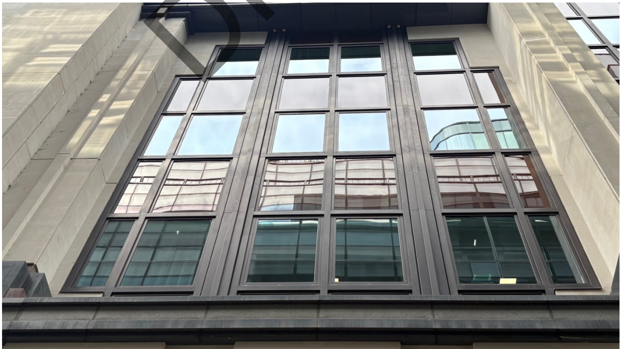
Photograph 6 – North elevation showing original infill area of curtain walling.
