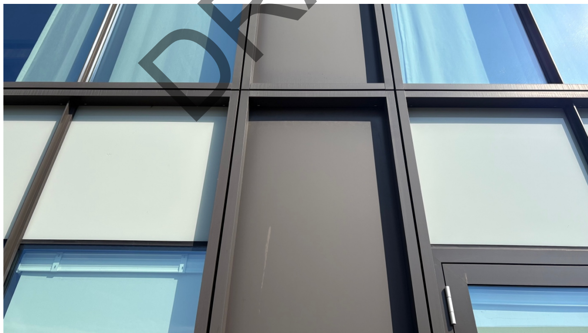
Photograph 16 – Close view of the 2017 installed curtain wall at Level 8 & 9.
