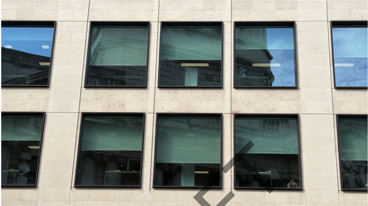
Photograph 3 – Front elevation showing the 2017 installed windows and Moleanos stonework.
