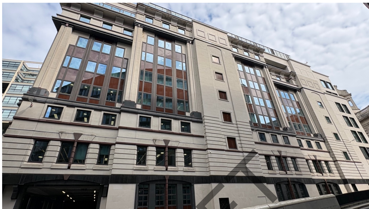
Photograph 7 – General view of the south elevation.
