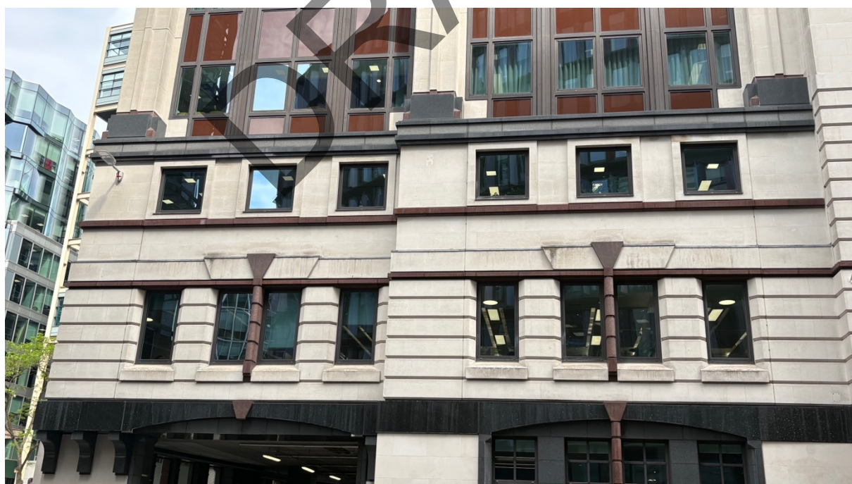
Photograph 8 – Part view of the south elevation showing the original stonework and windows.
