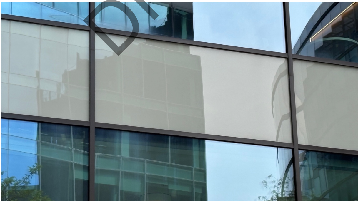
Photograph 12 – Glazed spandrel panel within the curtain wall as above.
