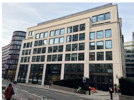
Photo of the front elevation, east facing.
