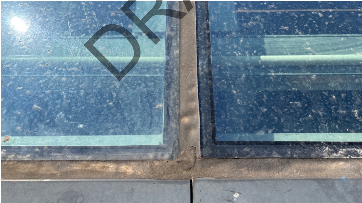
Photograph 18 – Close of the atrium roof silicone seals in a satisfactory condition.
