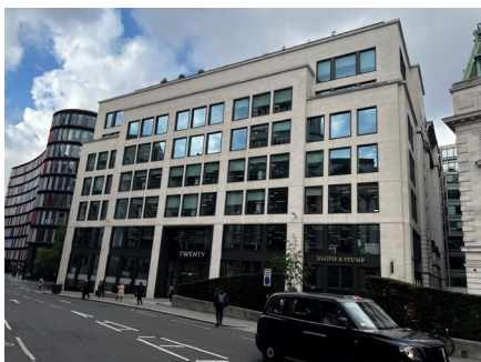
Photo of the front elevation.
