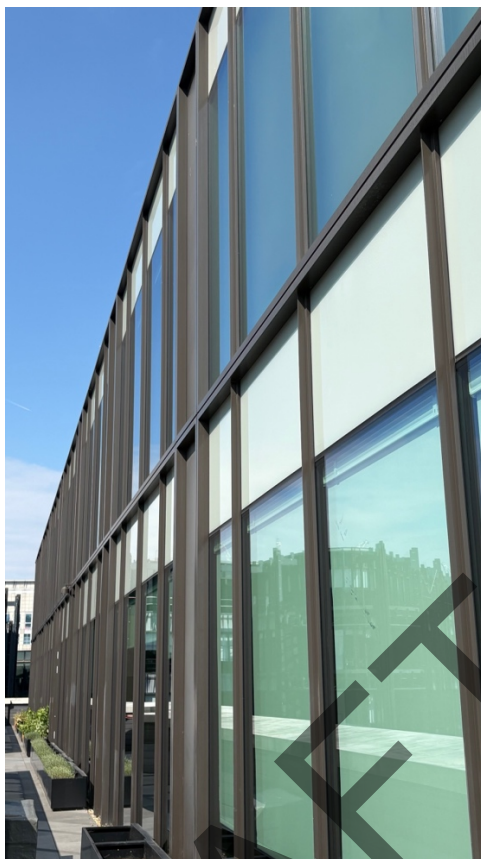
Photograph 15 – 2017 installed curtain wall at Level 8 & 9.
