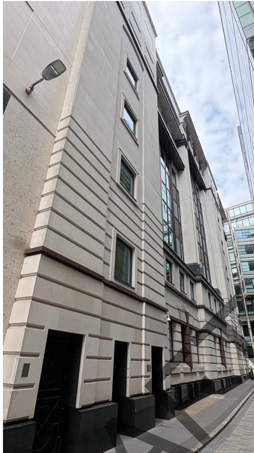
Photograph 5 – North elevation. (2017 stonework on the left and original stonework on the right)
