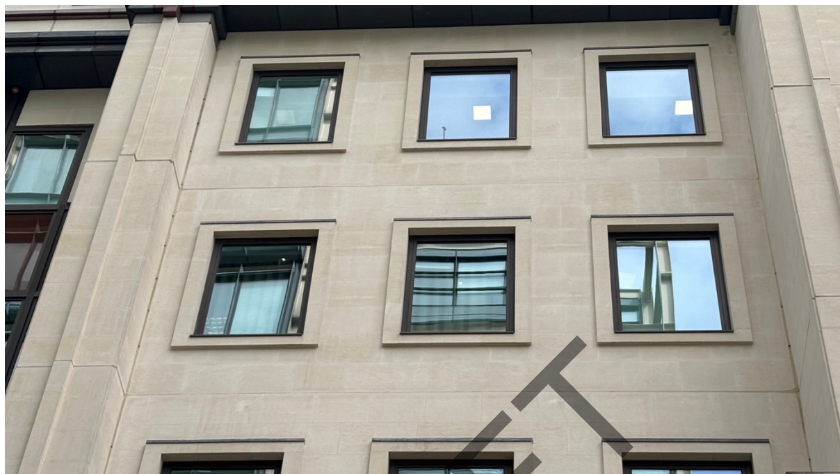
Photograph 13 – Rear west elevation showing the original stonework and windows.
