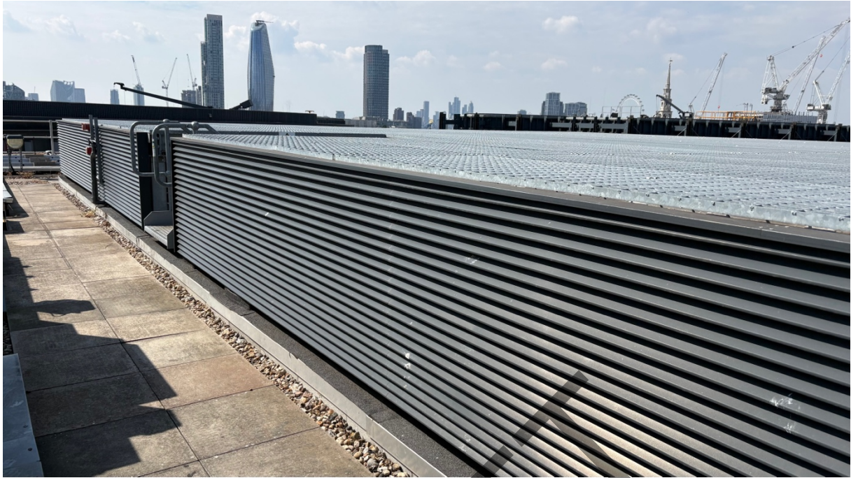
Photograph 19 - General view of the louvre blade open plant enclosure at roof level.
